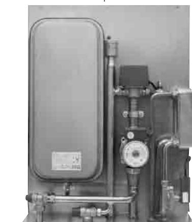
THE INLET AND OUTLET PIPES MUST BE CROSSED FOR THIS TO FUNCTION PROPERLY
